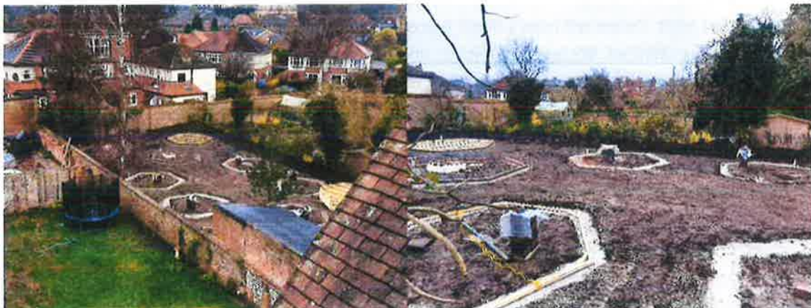
Photos of the rear at 6 St Georges Hotel (Photos taken 28 th November 2020)
